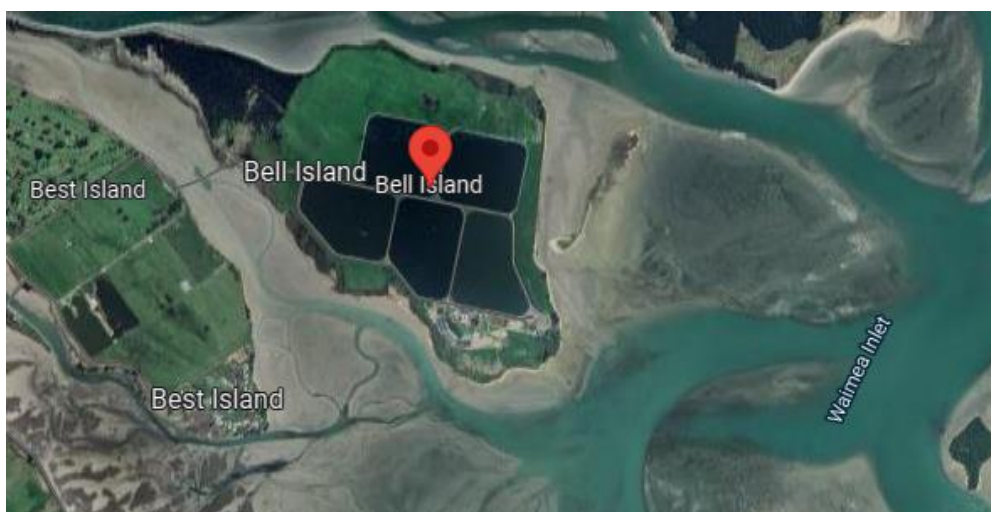
Figure 1 - Bells Island Treatment Facility
